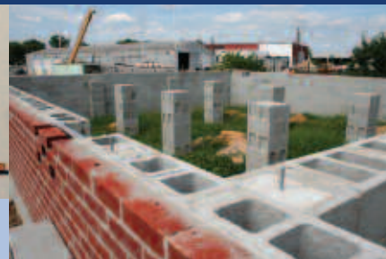
The foundation of the new Ruark Boatworks building, as of September 2009.
